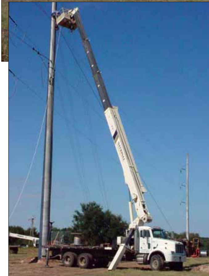
Above and left: Chapman Construction uses National Crane boom trucks fitted with manbaskets to help install power transmission lines.
