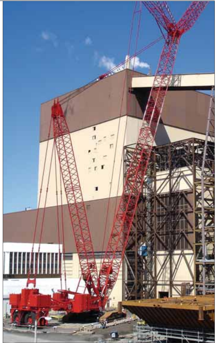
One of ALL Erection's Model 18000 crawler cranes.
