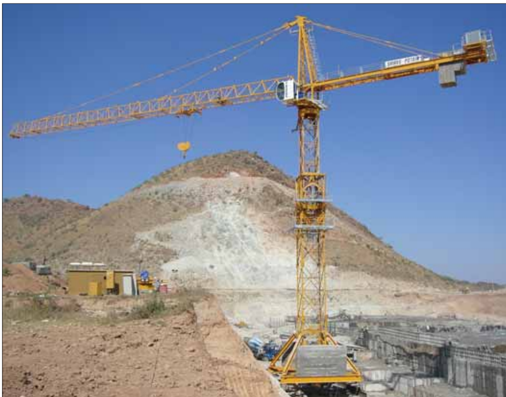
Potain tower cranes are a familiar sight on jobsites across India.
