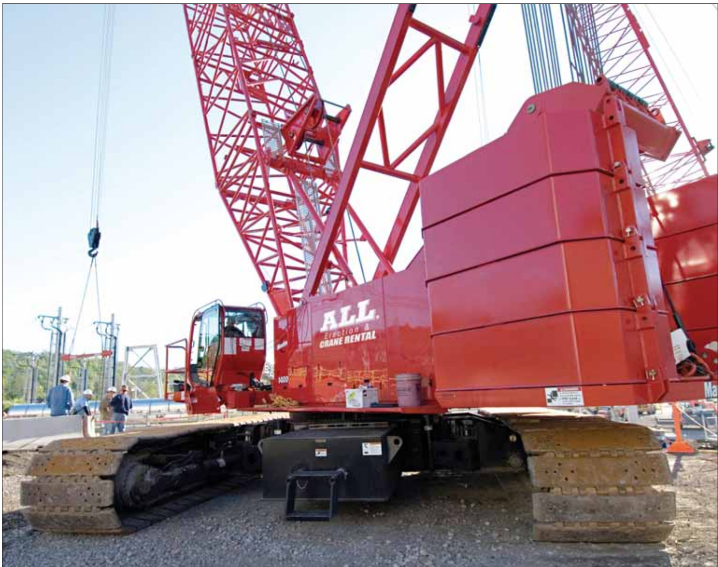
A Manitowoc crawler crane from ALL Erection fleet.
