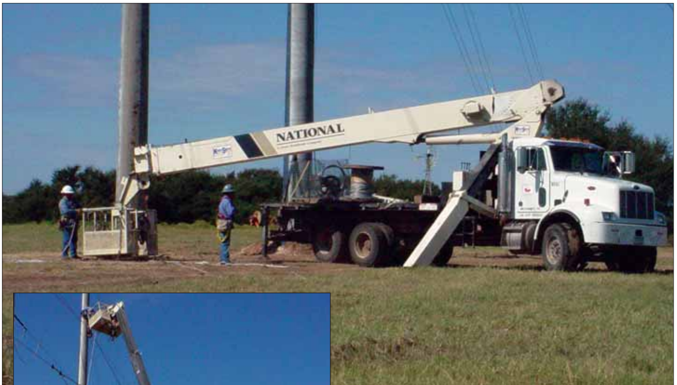
Above and left: Chapman Construction uses National Crane boom trucks fitted with manbaskets to help install power transmission lines.
