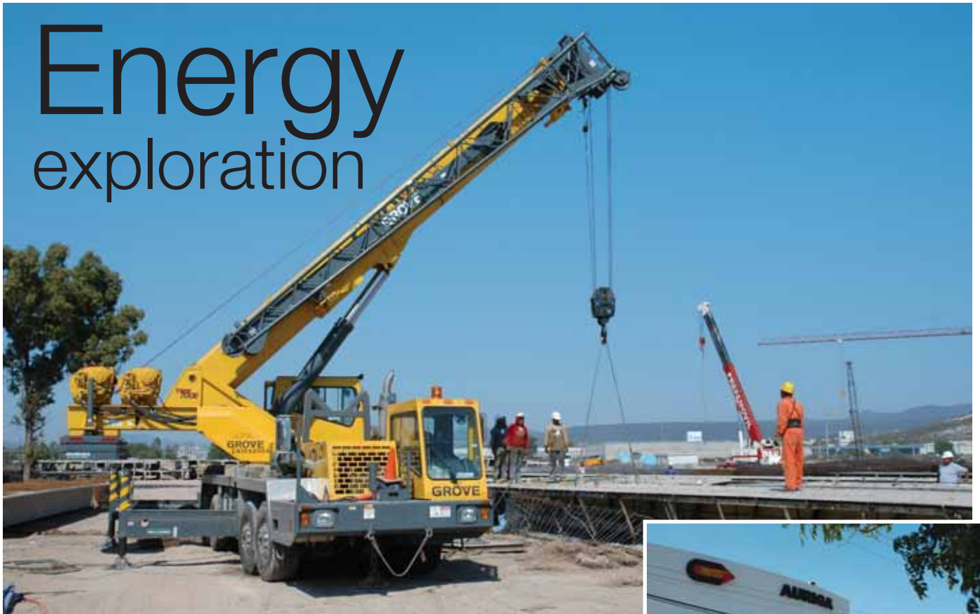
A Grove truck crane from the Auriga fleet in action.
