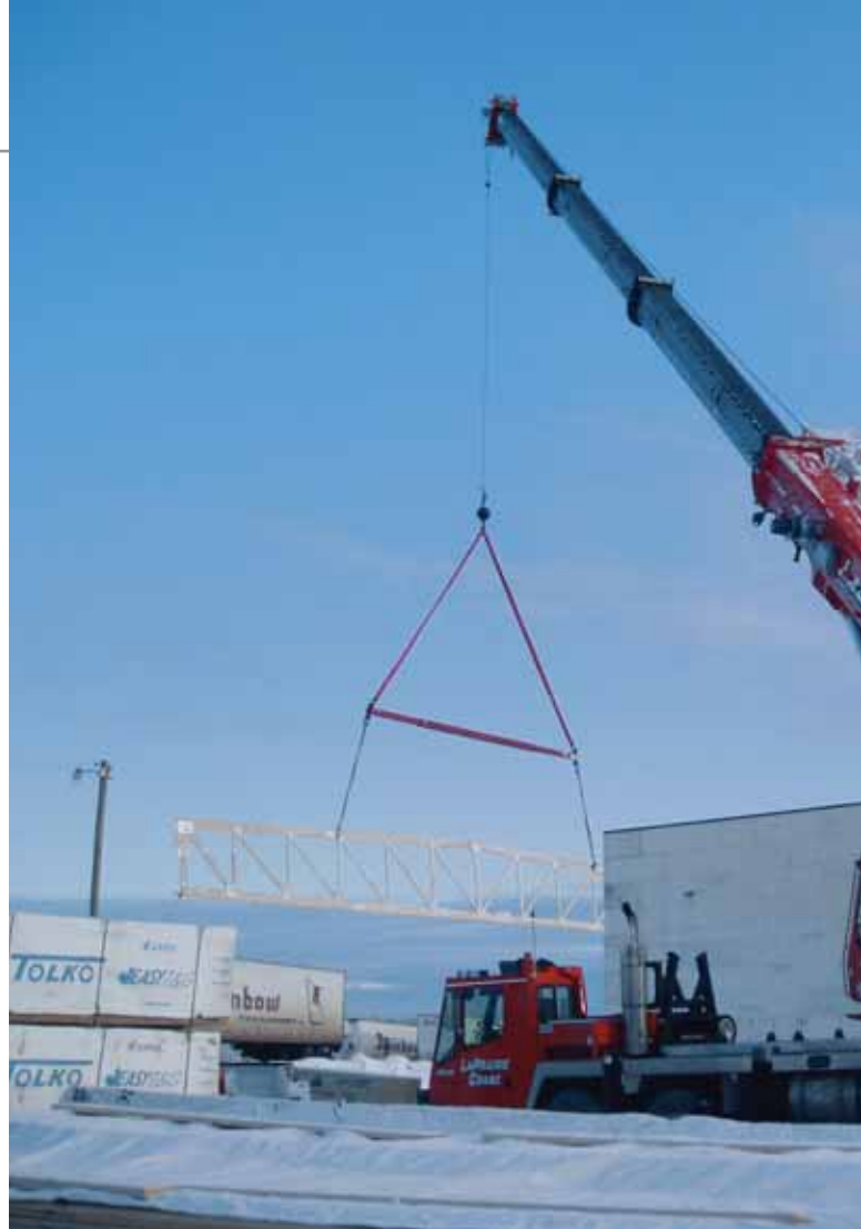
LaPrairie's TMS900E performs a variety of on-site lifting duties.
