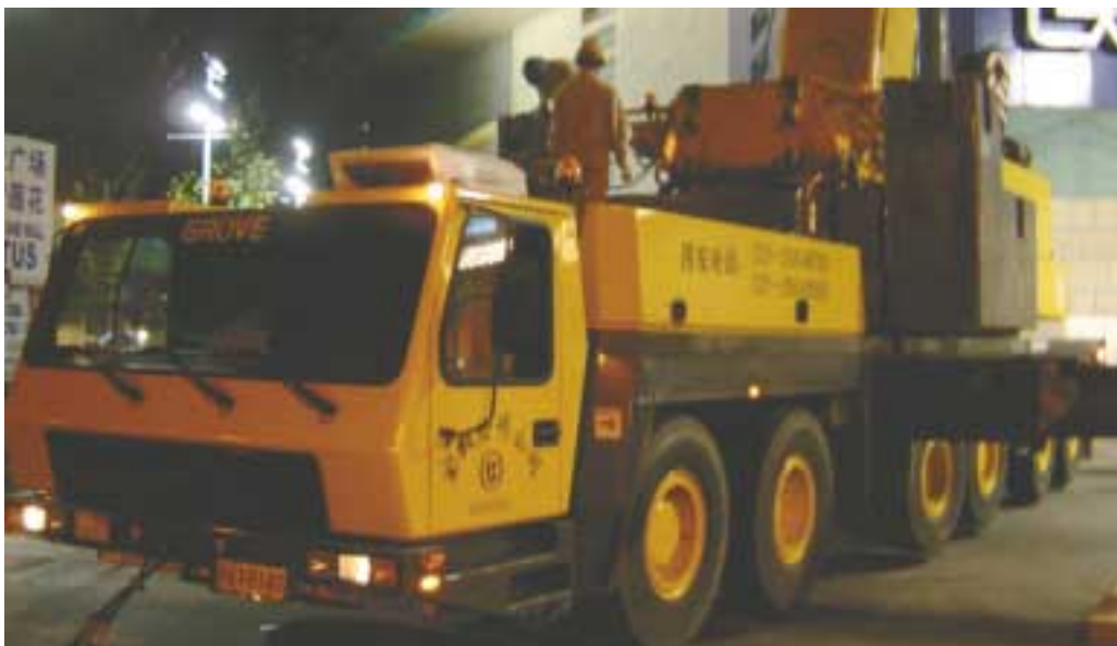
The crew from Baosteel worked through the night.
