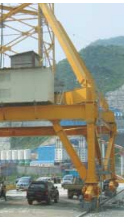
The rail portal on which the MD 1800 is mounted.
