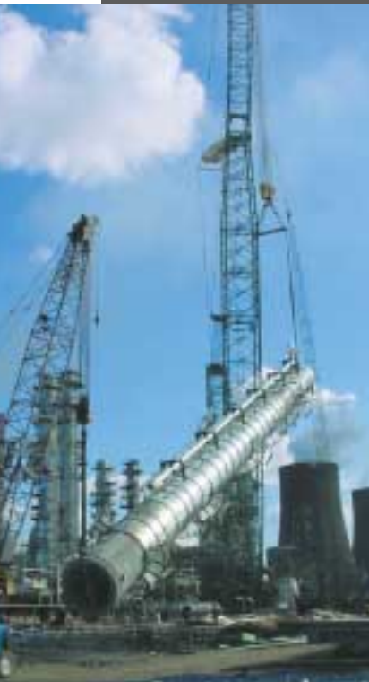
Pictured is a Model 1200 RINGER from Manitowoc Cranes positioning what is believed to be the tallest column ever raised by a single crane in the southern hemisphere. The crane, which is owned by chemical and fuel giant Sasol, made the lift at the company's oil-from-coal plant and refinery in Secunda, South Africa. Total length of the column is 111 m (364 ft) and it weighs 555 t (612 US t). It was lifted at a radius of 28 m (92 ft).
