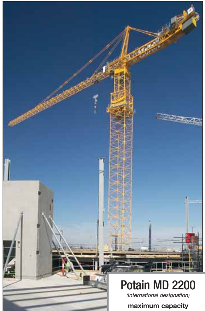
The Potain MD 2200 is thought to be the largest top-slewing tower crane ever put up in Australia.
