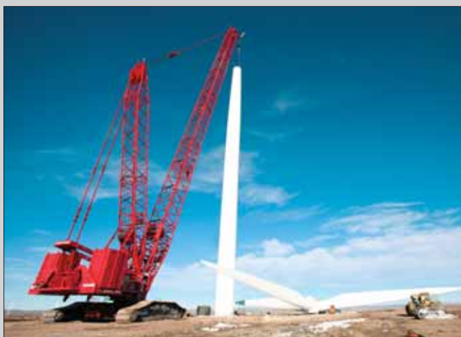
Each wind turbine takes approximately 14 hours to erect.
