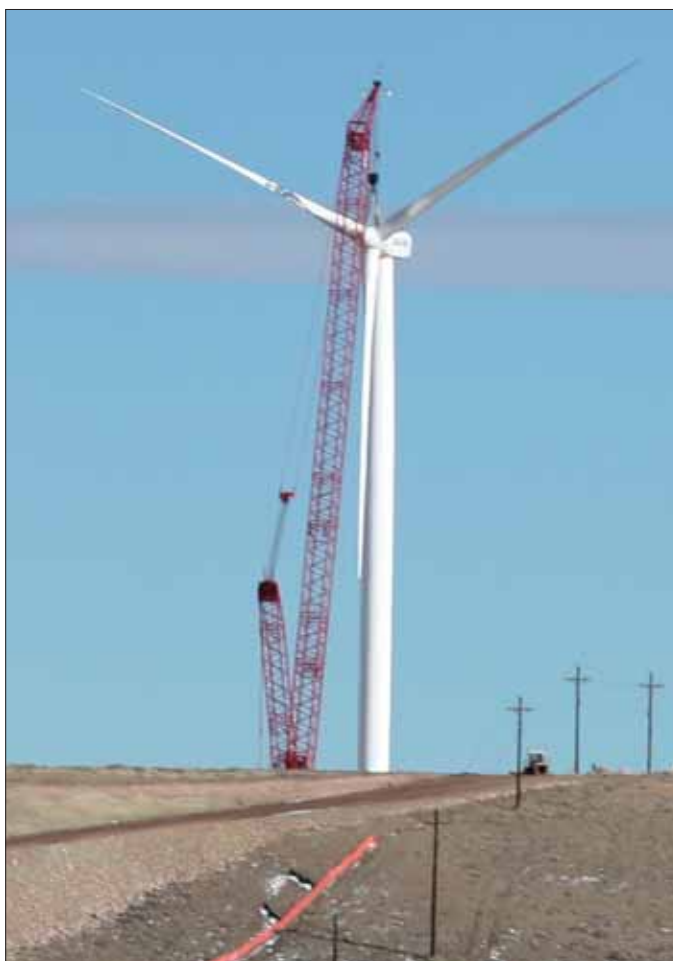
Mullen's Manitowoc Model 18000 crawler helps install the rotor on a 266 ft (80m) wind turbine in Fort Bridger, Wyoming.
